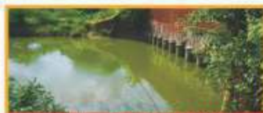
Gabion Retaining Wall
