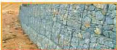
Gabion Retaining Wall
