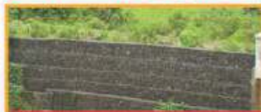
Gabion Retaining Wall
