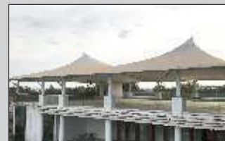
TENSILE STRUCTURE & RESIDENCY CLUB, KOLHAPUR
