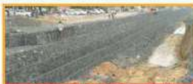
Gabion Retaining Wall
